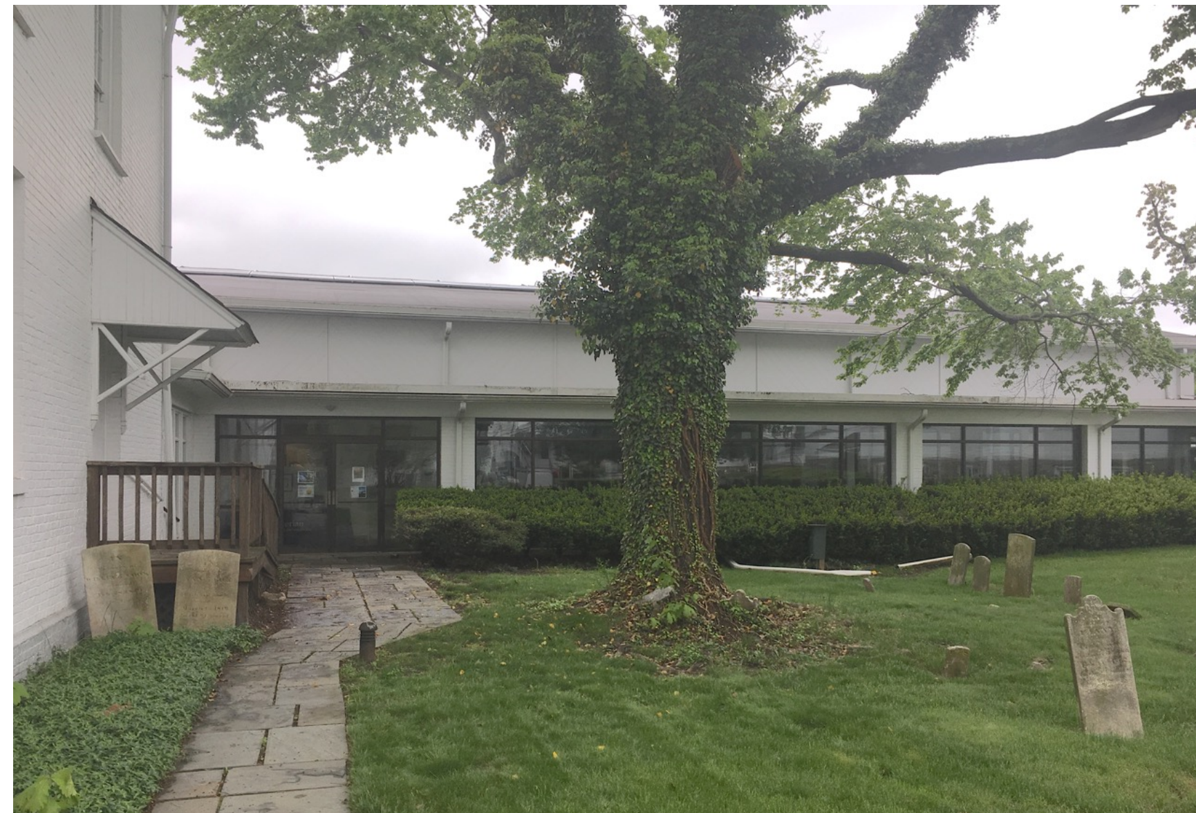
2 EXISTING VIEW FROM MAIN STREET
