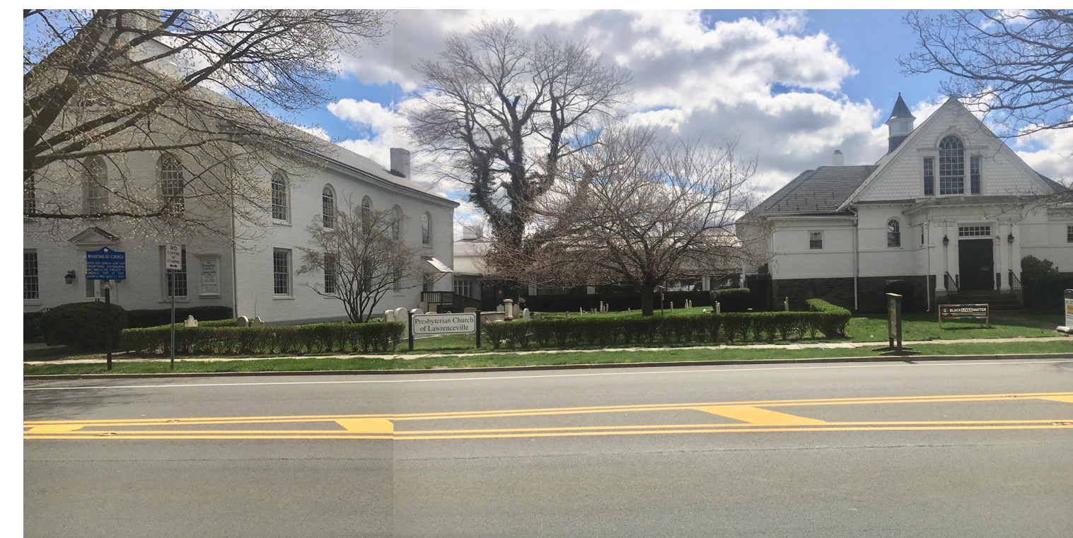
3 EXISTING VIEW FROM MAIN STREET
